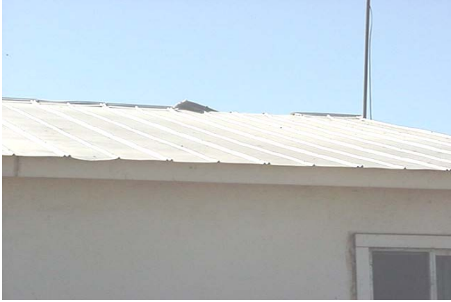
Metal roof damaged and leaking badly
