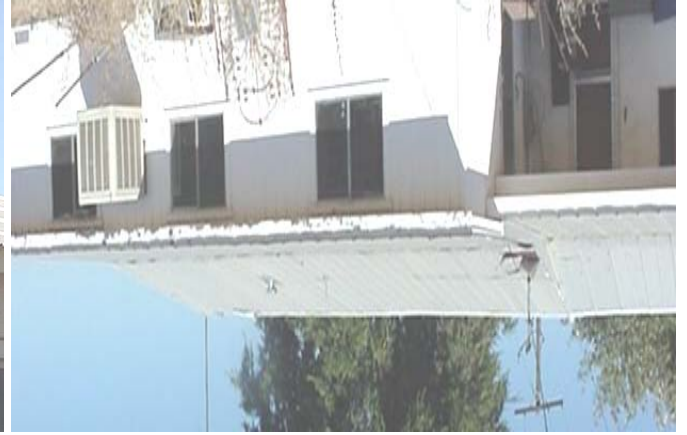
Metal roof damaged and leaking badly
