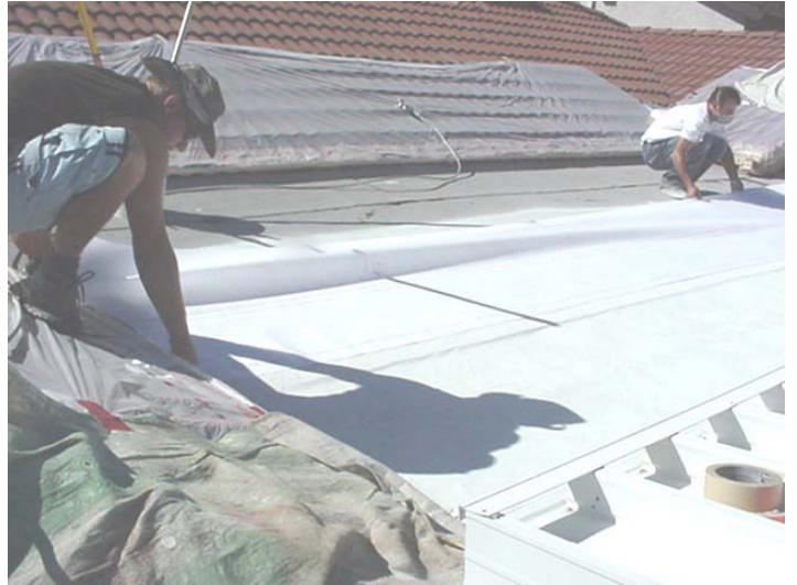
Embedding the cloth into the bottom coat with rollers
