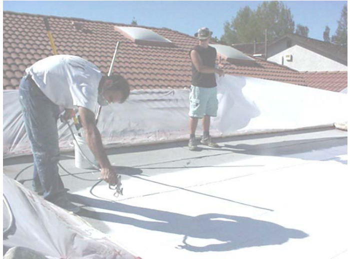
Spraying bottom coat on mineral capsheet roofing then 'Flying In' the roofing cloth
