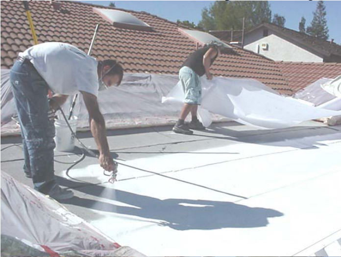
Spraying bottom coat on mineral capsheet roofing then 'Flying In' the roofing cloth
