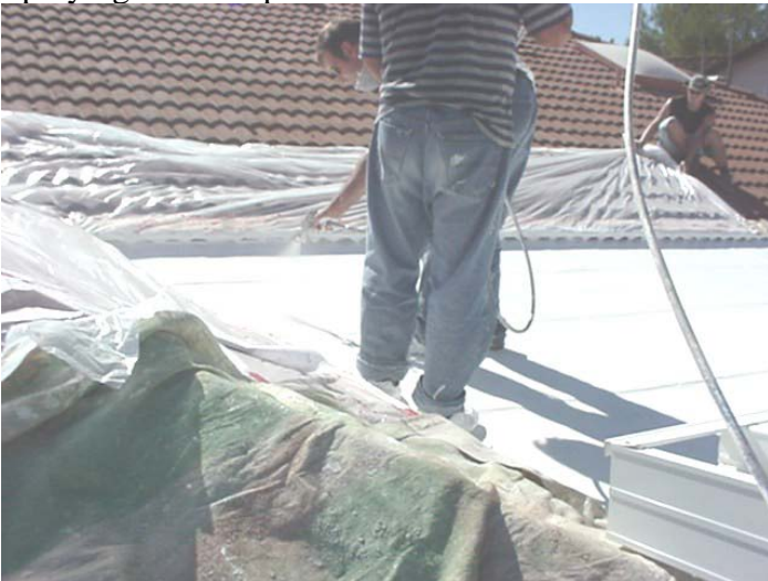
Spraying on the top coat of Cerama-Tech
