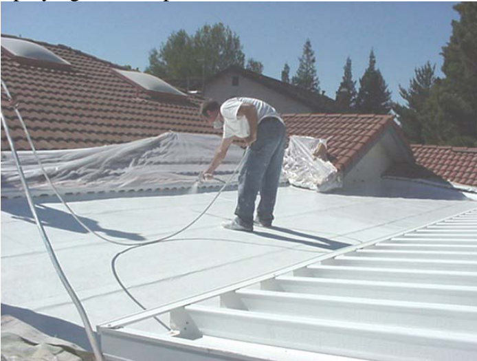
Spraying on the top coat of Cerama-Tech
