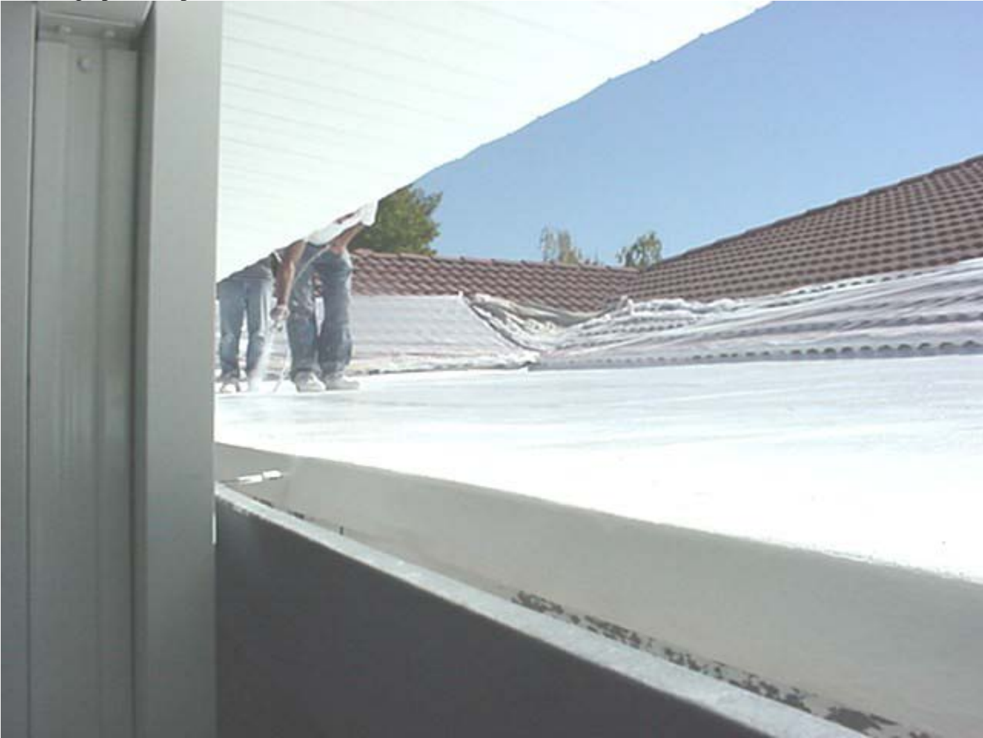
Finishing up with top coat.
