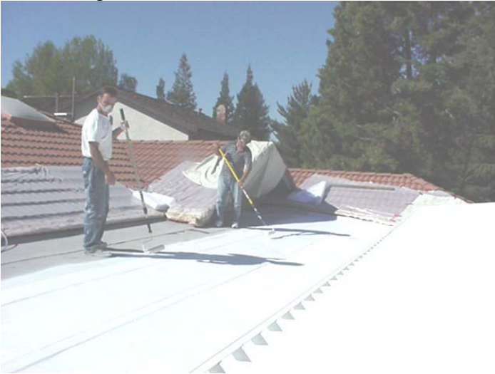
Spraying on the top coat of Cerama-Tech
