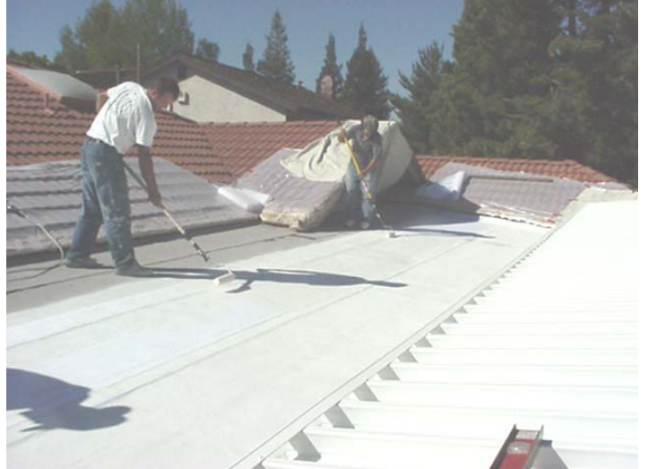
Embedding the cloth into the bottom coat with rollers
