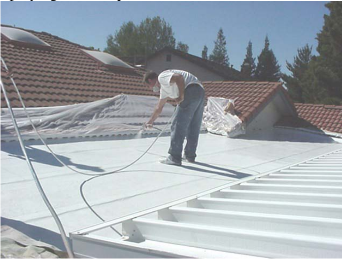
Spraying on the top coat of Cerama-Tech
