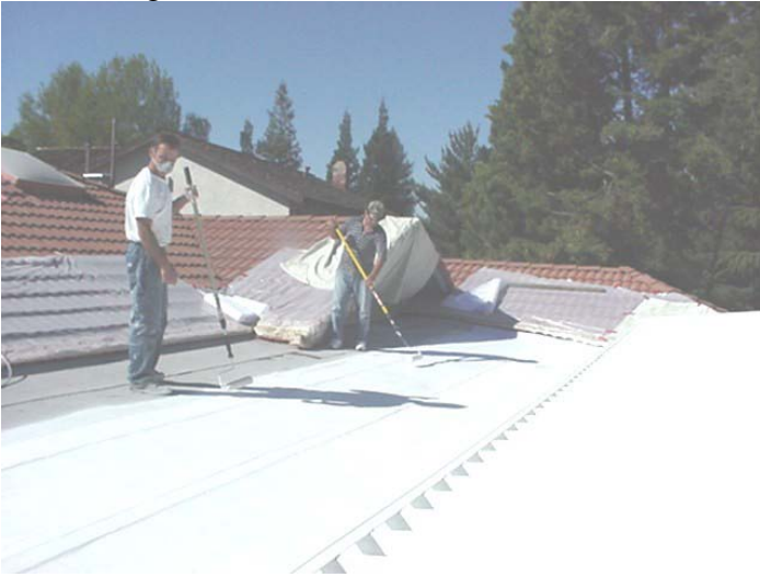
Spraying on the top coat of Cerama-Tech
